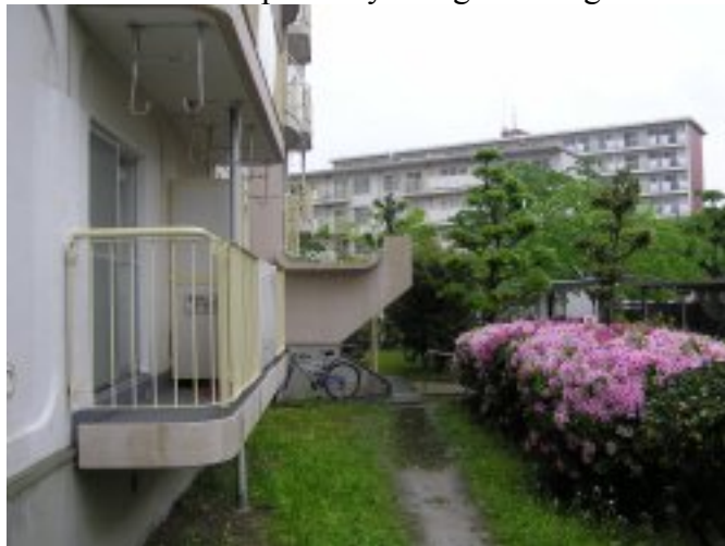
Figure 4-7: Apartments, Nisshin, suburb of Nagoya (Aichi Prefecture) These apartments are within walking distance of Nisshin Station.
