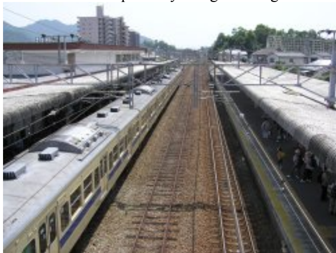
Figure 4-11: Miyajimaguchi JR Station, suburb of Hiroshima (Hiroshima Prefecture) Note the tall apartment buildings near the station. This is the JR station nearest Miyajima Island. Miyajima is famous for its water torii gate and Itsukushima Shrine.
