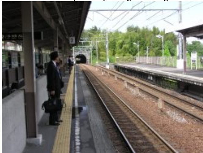
Figure 4-3: Nisshin Station (looking west), suburb of Nagoya (Aichi Prefecture)
