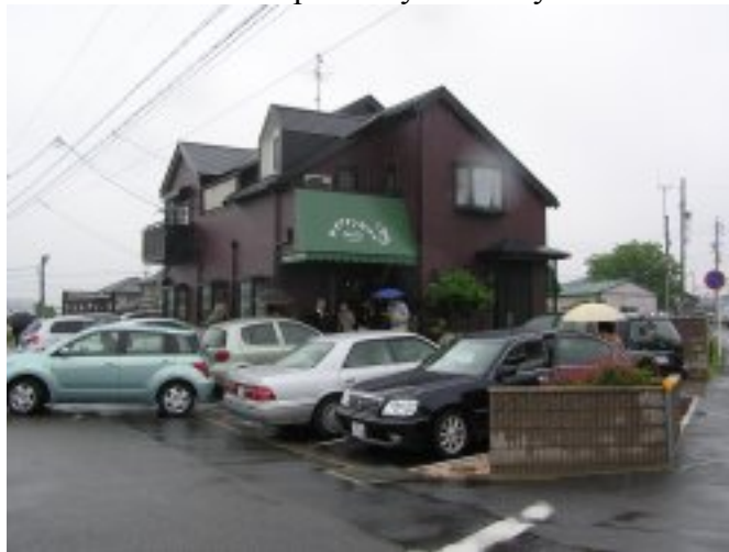
Figure 4-19: Shell Tea Restaurant, Togo, suburb of Nagoya (Aichi Prefecture) Source: photo by Craig R. Laing
