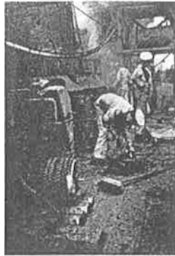
Damage to the deck of HMS Chester sustained during the Battle of Jutland.
